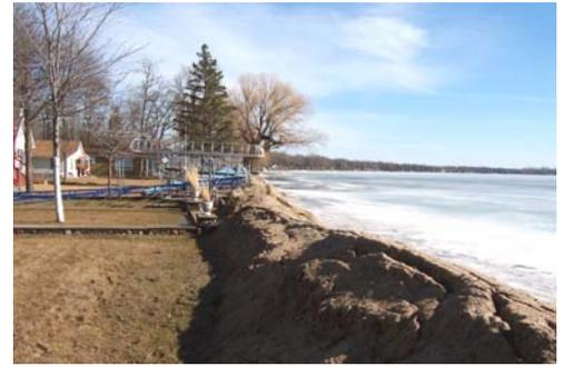
Remember, a minimum of an eight-inch berm parallel to the water's edge is required in order to prevent shoreline runoff to the lake.
